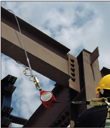
Example of a Self-Retracting Lifeline used with a Temporary Anchor
