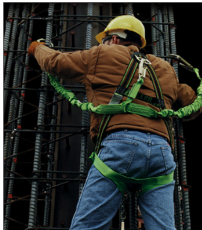
Example of a Shock-Absorbing Lanyard in use
