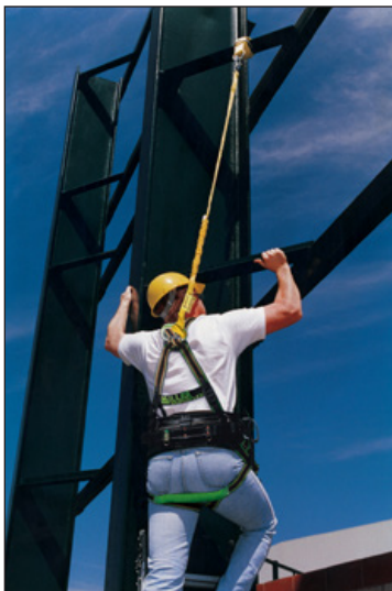
Example of a Restraint Lanyard in use
