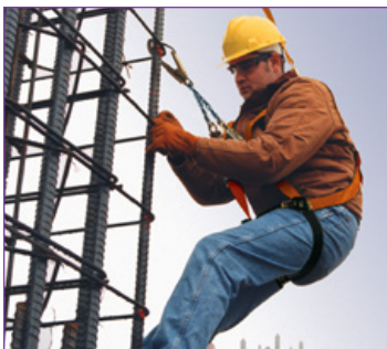
Example of Fall-Arrest System
