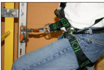
Example of Work-Positioning System
